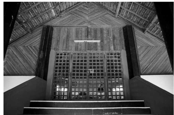
(Top) Software Campus for CA India Technologies Pvt Ltd, Hyderabad; (Above) Kalakshetra - Centre for Performing Arts, Chennai
